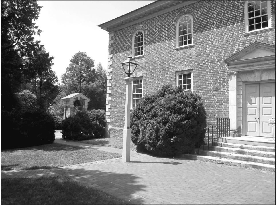
Pohick Episcopal Church, (circa 1774) designed by George Washington, and Parish Church of George Washington, George Mason and William Fairfax, Vestrymen.
